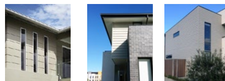
Lightweight Cladding types - horizontal panel
