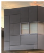
Lightweight Cladding types - flat panel
