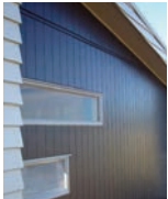
Lightweight Cladding types - vertical panel
