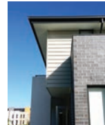
Lightweight Cladding types - horizontal panel
