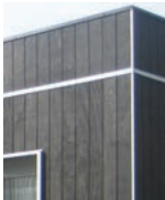
Lightweight Cladding types - vertical panel
