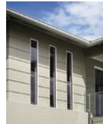
Lightweight Cladding types - horizontal panel
