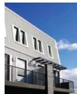
Lightweight Cladding types - corrugated and battened
