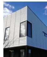
Lightweight Cladding types - corrugated and battened
