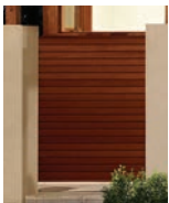
Lightweight Cladding types - timber
