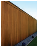
Lightweight Cladding types - timber
